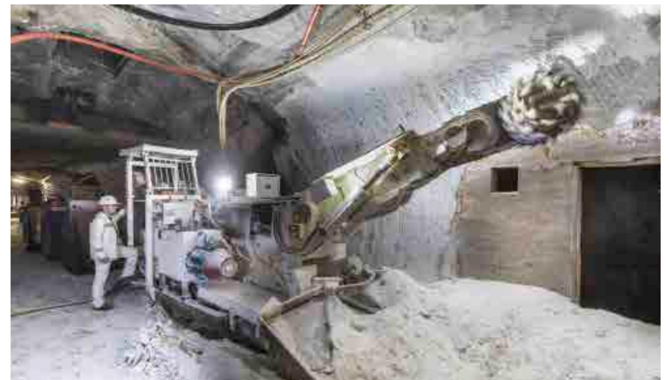
Re-trimming for the installation of a ventilation gate (Morsleben repository)
