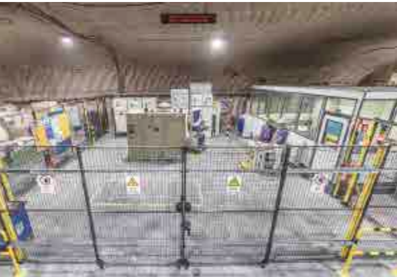
Setting up a test field for 5 kilovolt stations
