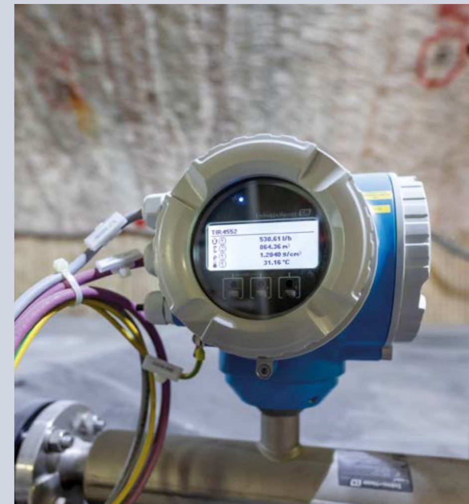
Asse mine: A new device for measuring flow rate, density, and temperature at the main intake point on the 658 m level
